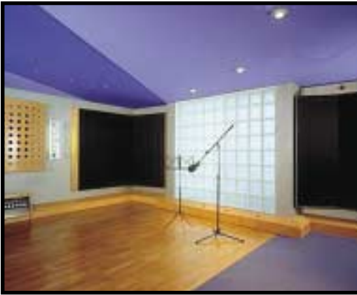
Live area using prefabricated Black Box for acoustic control.
