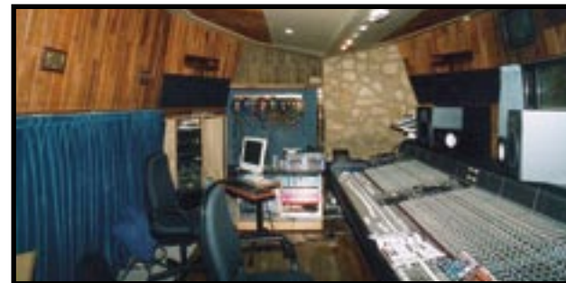
Fig. 2. Quadrophonic control room of the 1970s showing the two 'front walls' of a stereo room facing each other. Note front speakers are flush-mounted but the rear ones are mounted above the soffits of the machine alcoves — another source of asymmetry.
